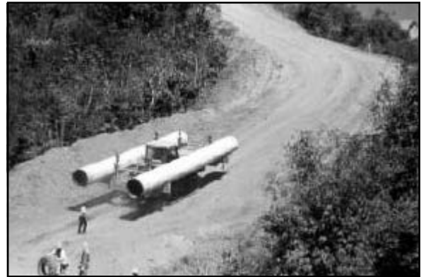
Building the pipeline
