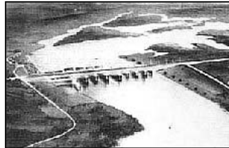
The Pak Mun Dam
